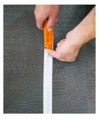
Overlap 2 sheets of flooring so the pattern repeat of two side-by-side squares is 15 cm. Cut so one square is about 7.5 cm.
