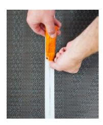
Overlap so the pattern over two stripes are about 6 cm. Cut so the stripe is around 3 cm.
