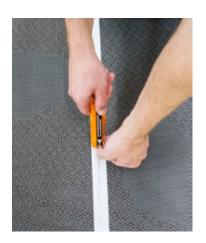
Overlap 2 sheets of flooring 4 cm and double cut. Make sure do not cut in the big dots..
