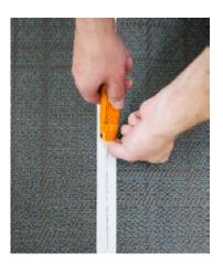
Overlap the entire smooth section over the mottled. Cut so that the smooth section is around 1.5 cm. The width of the mottled section is of secondary importance.
